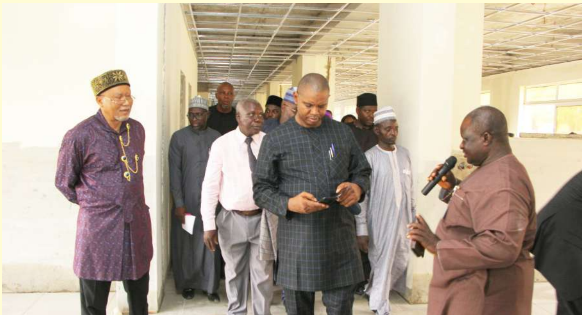
Engr Bala Mangut, taking the Board Members on an inspection tour of the Mental Health Block
