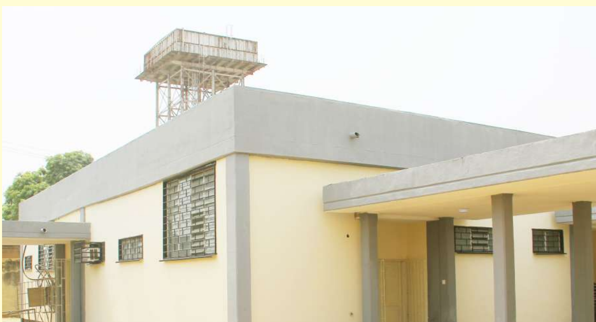
The Renovated and Equipped Laundry Department
