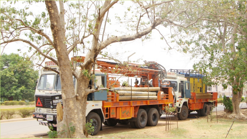
Visit to the New Water Reticulation sites within the Hospital.
