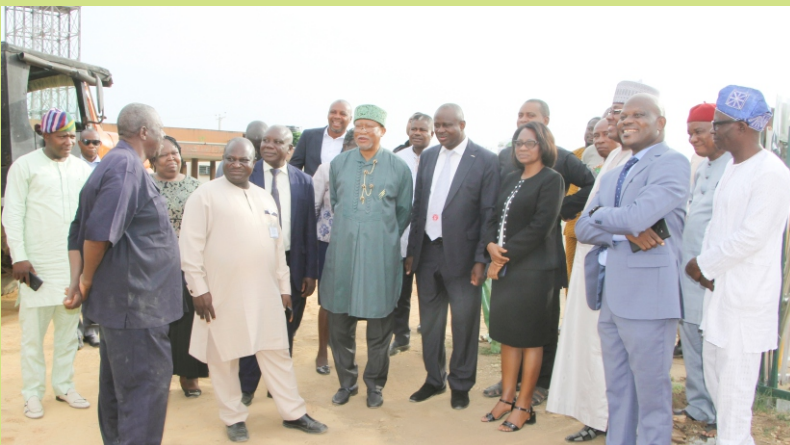
Board Members visit to the NLNG Center Construction Site.
