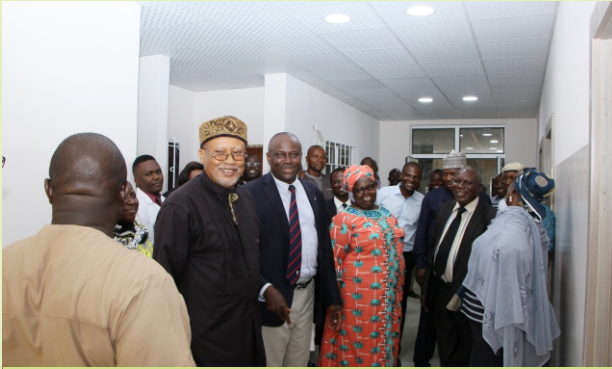
The Board led by its Chairman, Dr. Sam Sam Jaja inspecting the restructured and renovated Administrative Building.
